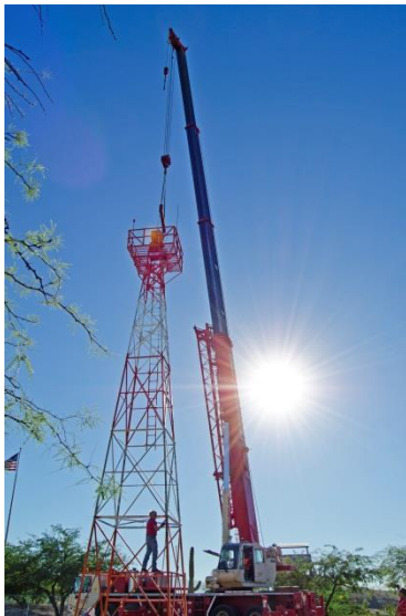
PASMBeaconCrane.jpg = crane moving the beacon to its new location near Valencia Rd. during the early morning. Photo by Andrew Boehly
